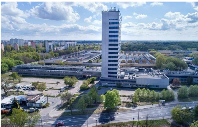
CeMat & PKO BP office building
