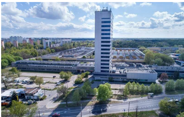
CeMat & PKO BP office building
